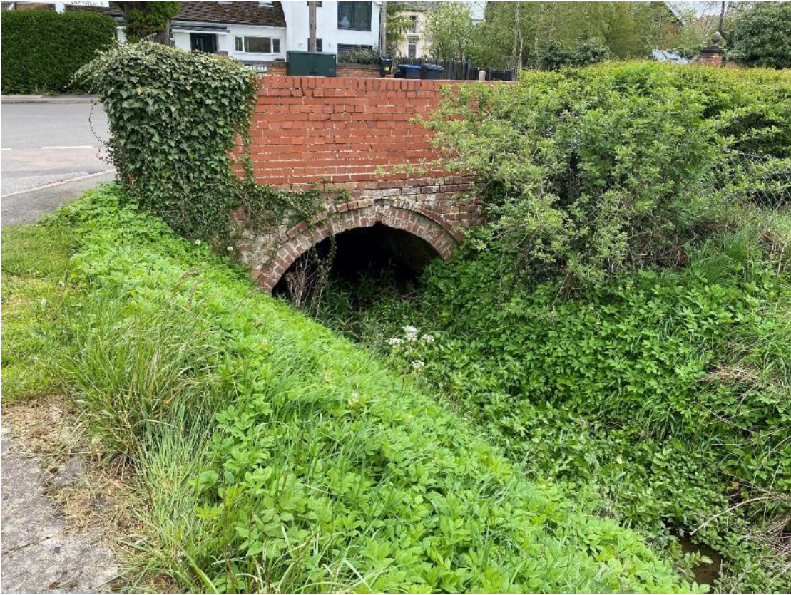
Entrance to Yelvertoft Brook culvert, south of High Street
