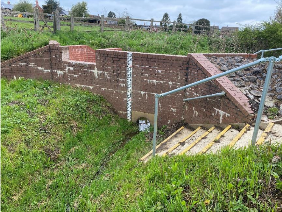
Flood Alleviation Scheme on Yelvertoft Brook, south of High Street.
