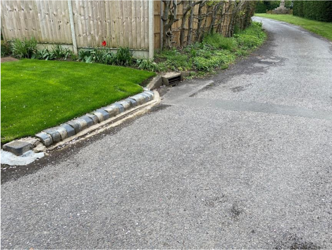
Access to Yelvertoft Brook culvert, Swinnertons Lane
