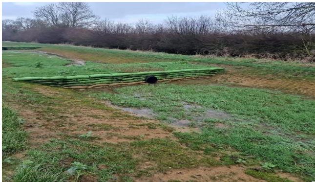
Swales have drained and are gaining in grass cover
