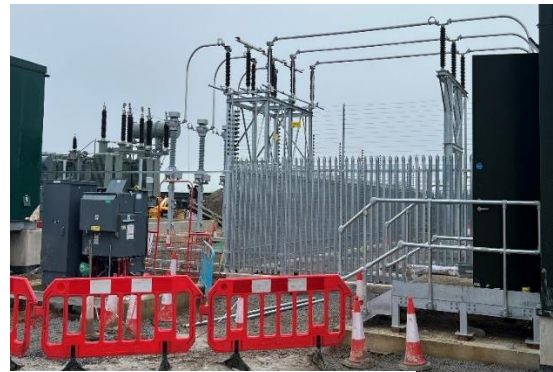
Grid connection works are ongoing
