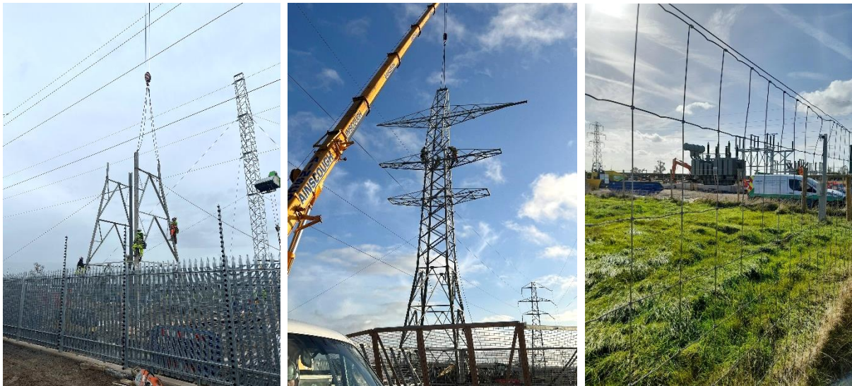
Grid connection works
