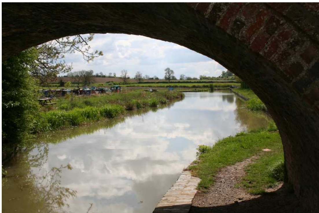
▲ Grand Union Canal at bridge 18 (listed building) - Yelvertoft Marina is on the left
