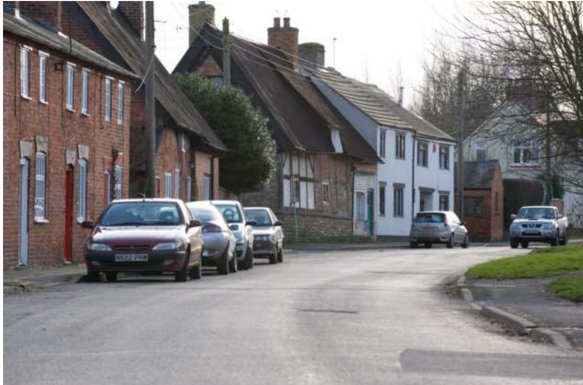
▲ Elkington Road showing two listed buildings between terraced cottages.
